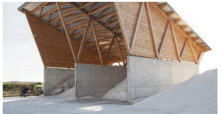
Mass timber panels being installed at Evergreen
