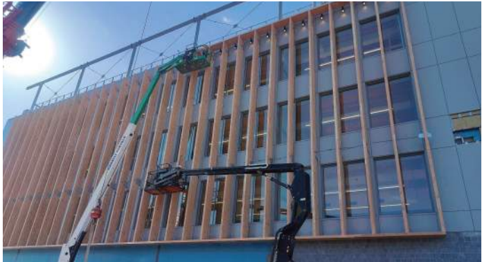
Mass timber panels being installed at Evergreen
