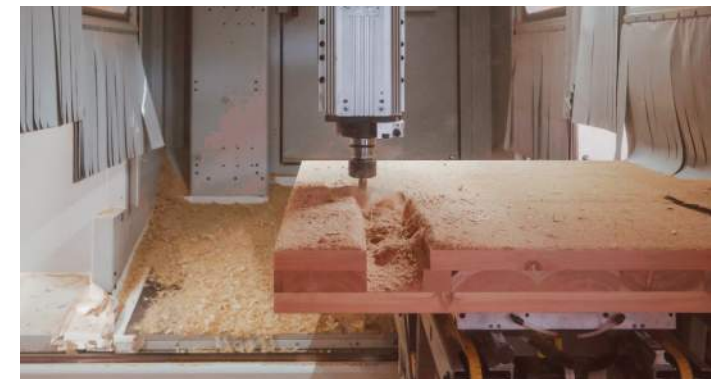
Mass timber panels being installed at Evergreen Charter School, designed by MHA.
