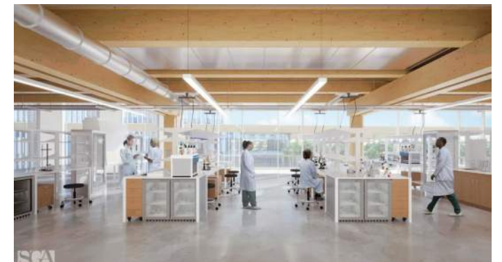
Mass timber panels being installed at Evergreen
