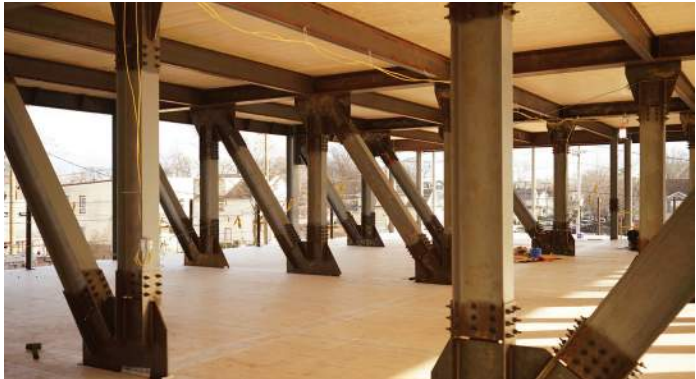
Mass timber panels being installed at Evergreen
